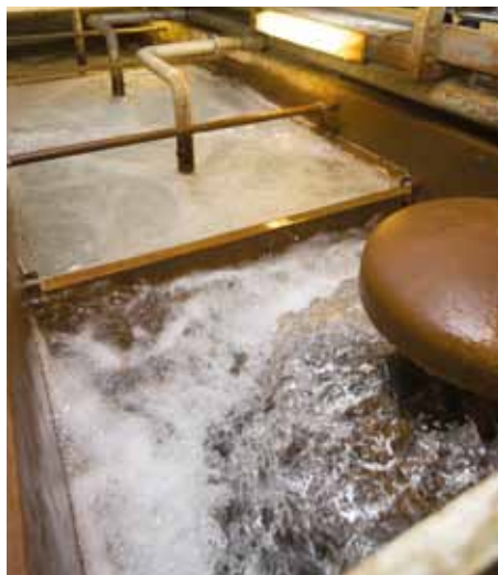
Groundwater aeration with the help of air bubbles.
