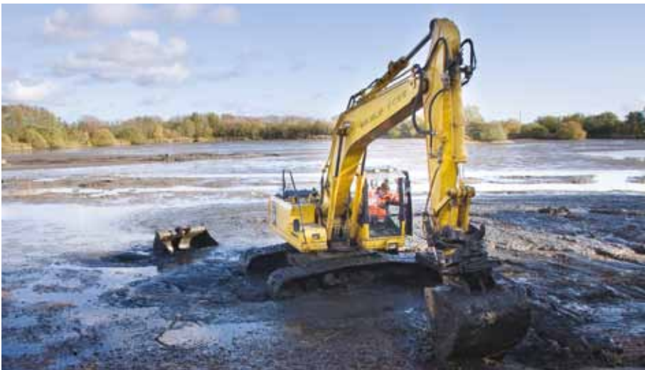
A storm water pond at Tranbjerg being emptied of sludge and re-established as a recreational area.
