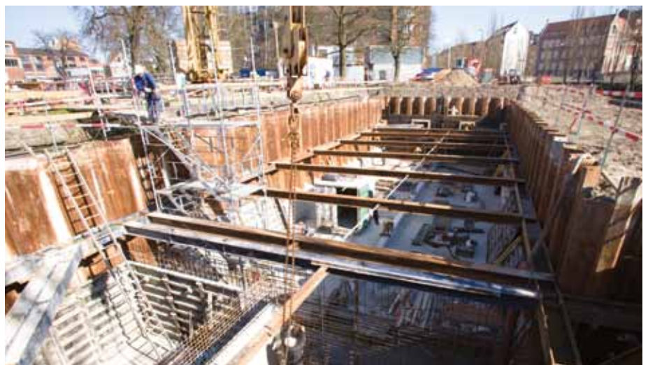
Building a retention tank at Mølleparken.
