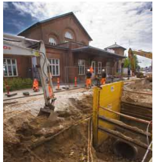
Excavation in connection with sewer pipe replacement.
