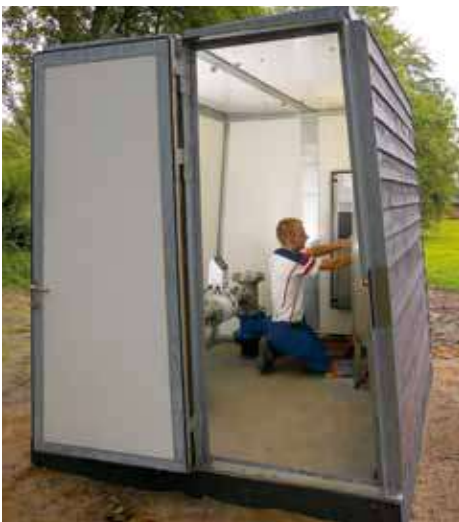
A well cabin under construction at a groundwater well.
