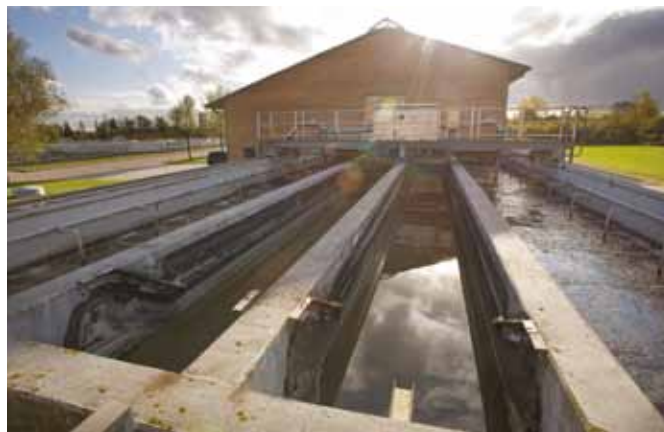
Sand and fat separation ponds at Egaa Waste Water Treatment Plant.
