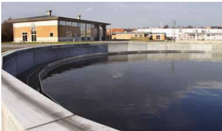
Clarification pond at Aaby Waste Water Treatment Plant.
